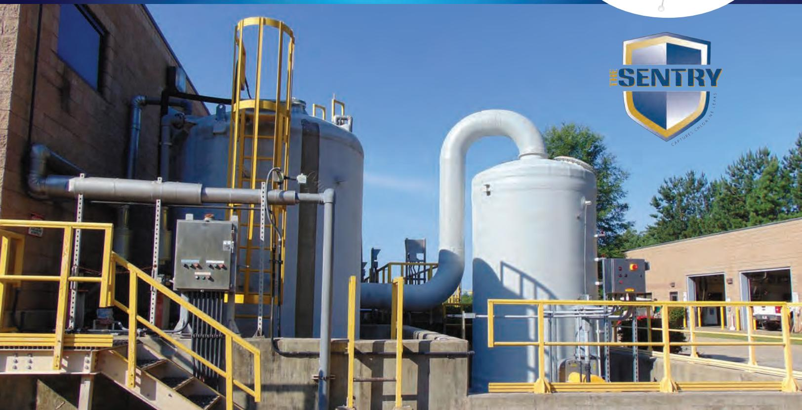
PureAir Filtration's Sentry™ Emergency Gas Dry Scrubber is the best line of defense against toxic gas leaks at facilities that use gases that could be harmful to health and safety if released; such applications include chlorine tanks used at water treatment plants. With only one moving part, the Sentry™ is safer, more reliable, and easier to operate than old fashioned wet scrubber systems, also requiring less maintenance and costs.
