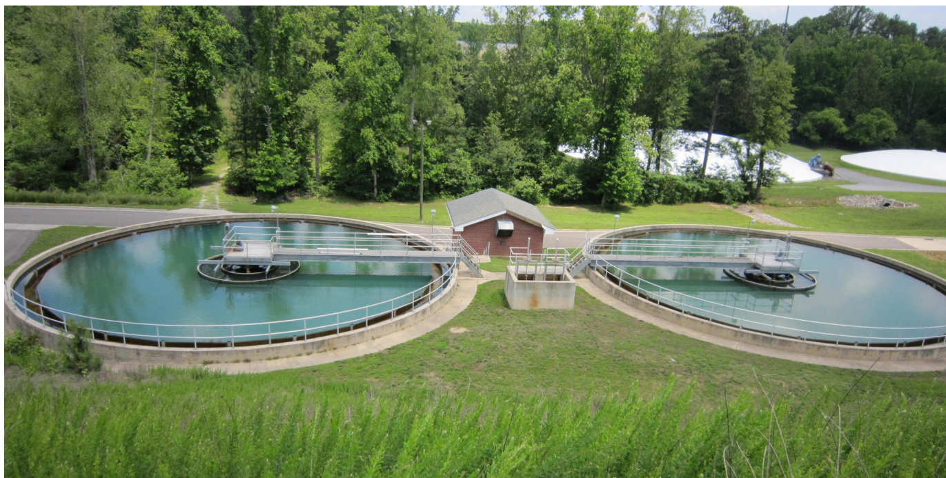
Water treatment site
