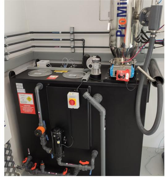
ProMinent's Pro Sat - Vac Fluoride Saturator System. Provides a safe & economic way of dosing fluoride into your water supply with ProMinent's Vacuum Loading System. To ensure dust free loading of 25kg sodium fluoride bags.
