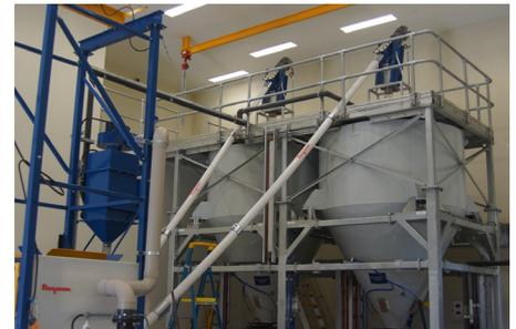
ProMinents Bulk Bag Sodium Silicofluoride (SSF) Feeder System. The ProMinent Silicofluoride Bulk Bag Preparation and Transfer System is variable concentration, constant transfer system; designed to maintain a constant level of fluoride in the fresh water being processed by the water treatment plant.
